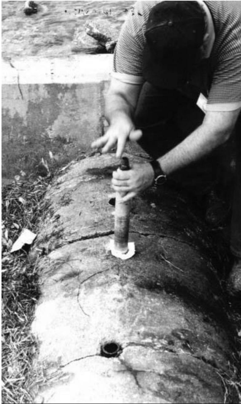
Figure 30. Site No. 7. End of San Jose Street. Low Tide. Core extraction. Evidence of pipe distress.
