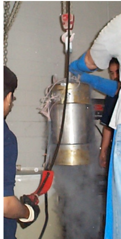
Figure 7.25 Cold trunnion taken out of the dewar.
