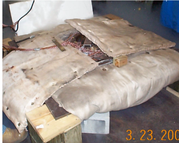
Figure 7.22 Induction heating coils for heating the hub-girder.
