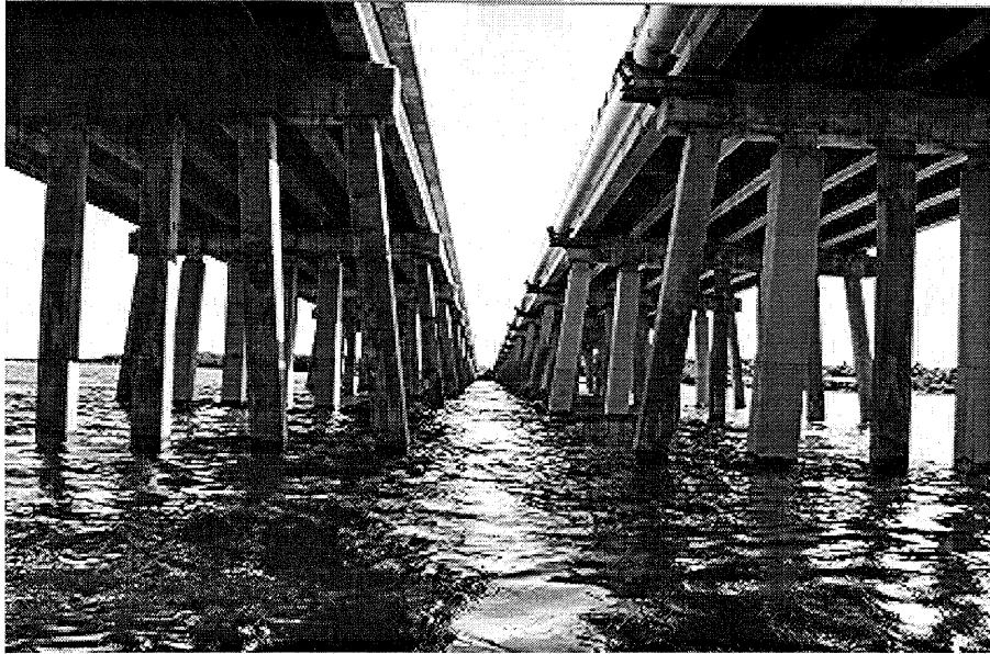
Figure I.4. Over water structure located on the Florida keys (South (right) and North (left) bound Bahia Honda Bridge built in 1969 and 1972 respectively).
