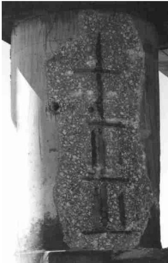
FIGURE 1 - Typical spall appearance (7MI)
