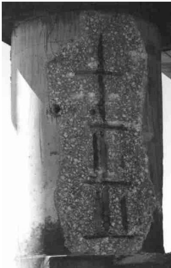
FIGURE 1 - Typical spall appearance (7MI)
