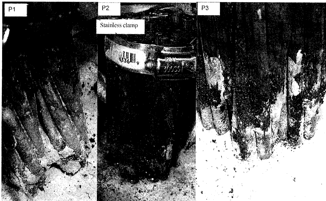
Figure 4. Rusting On Strands In P Series Assemblies At Day 308 (After Three Water Recharge Events) Severe air space corrosion on all three bundles. Slight grout/void interface rusting in P3. White grout residues left by bleed water.
