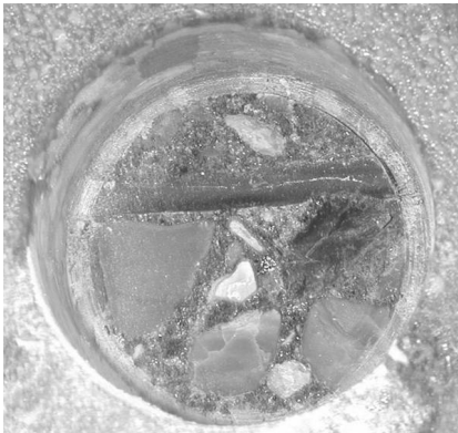
FIGURE 1- Exposed spiral wire, no corrosion. Pile H29-3.
