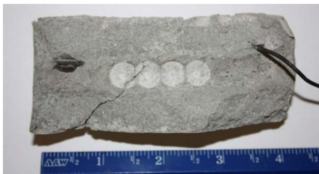
Figure 4: Drilled holes for the mortar collection at the rebar trace (scale in inches).
