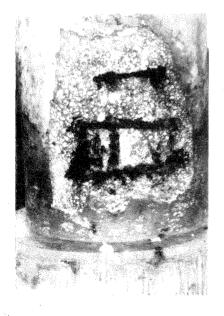
FIGURE 1 - General appearance of corrosion in a bridge column using epoxy-coated reinforcing steel.
