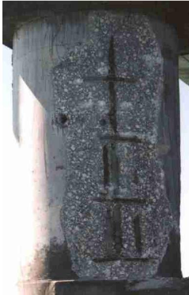
Figure 1. Typical Spall Appearance (7MI)
